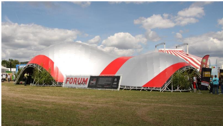
Figure 8. GFRP elastic gridshell for Solidays Festival [17]
