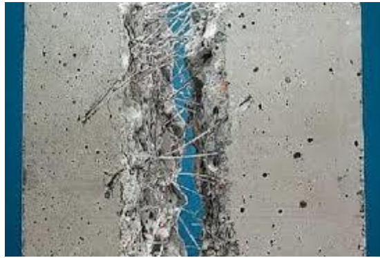
Figure 1. View of fiber concrete
