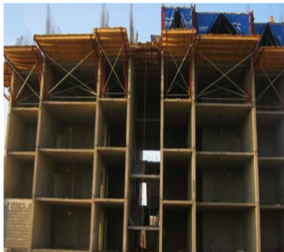
Figure 4. The execution sample of mass housing projects in Iran using modern tunnel molding technology
