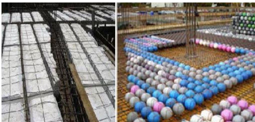
Figure 5. Images of Cobiax technology and the traditional technic of concrete joists and foam.
