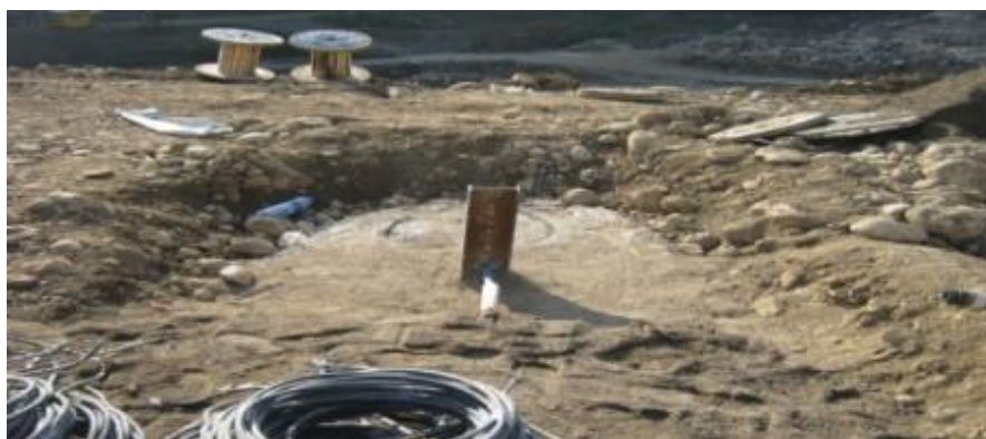
Figure 15. Fixed point at level of 175 m in Shahr-e-Bijar Dam
